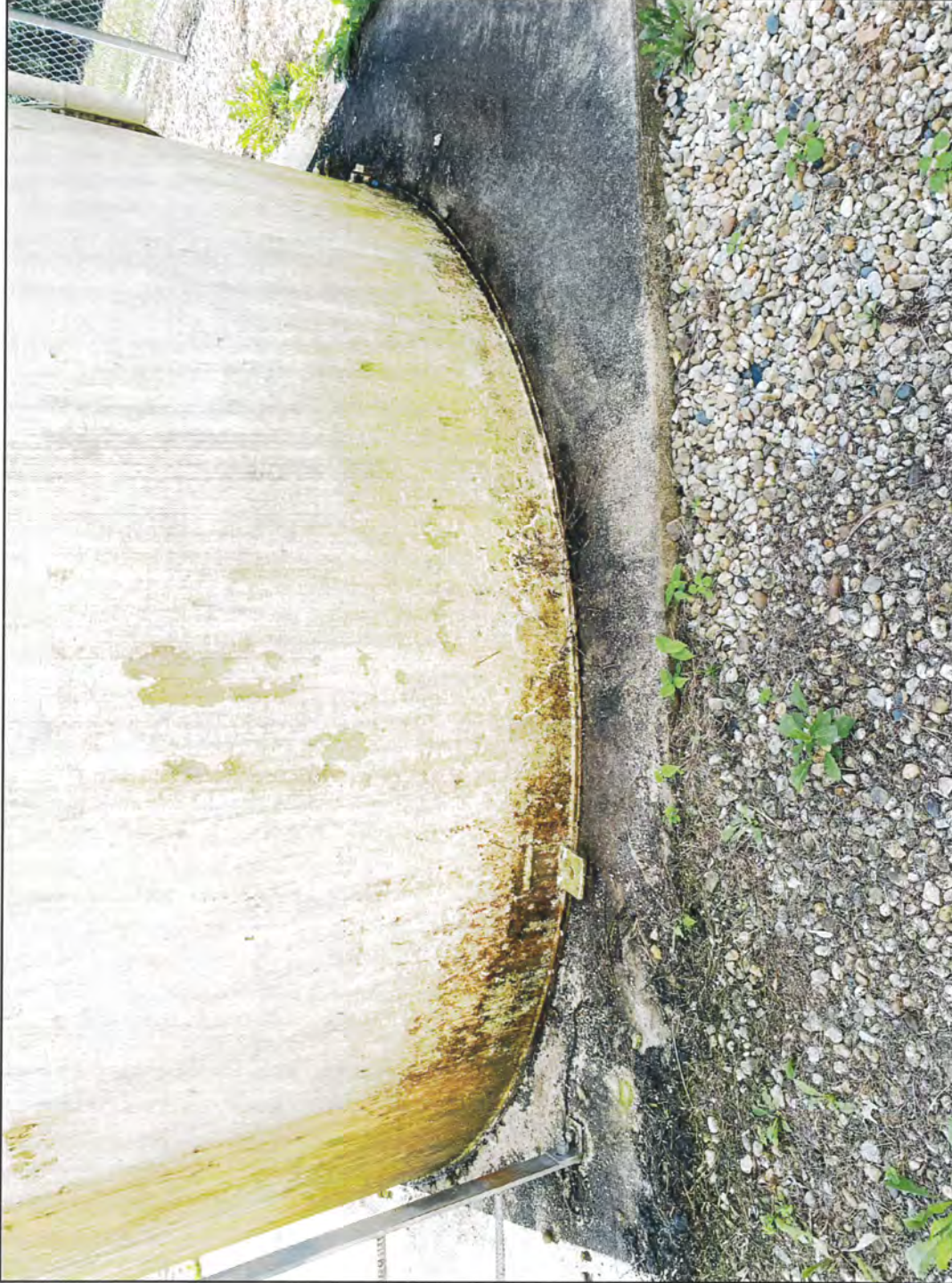
CHIME AREA OF AERATOR TANK
