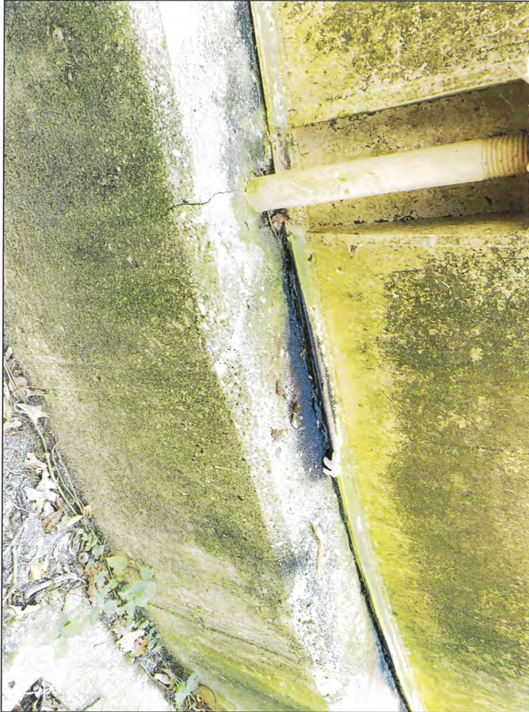
CHIME DAMAGE AND GROUT NEEDED (TYPICAL)
